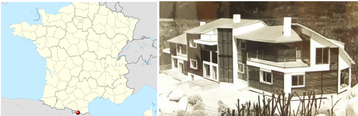
Figures : The solar house building Trombe-Michel and its location
