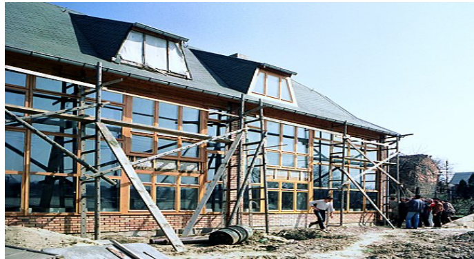
Figure : A building using Trombe wall as a passive solar strategy in Hopfgarten, Austria
