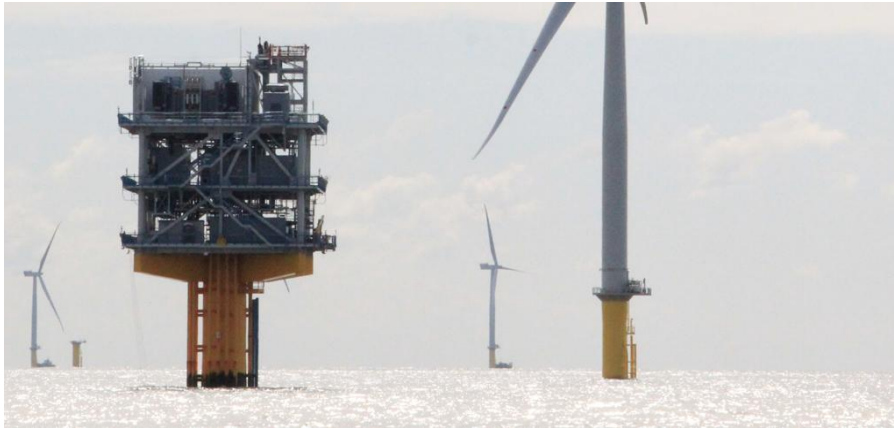
Illustration 11: Station de transformation offshore
